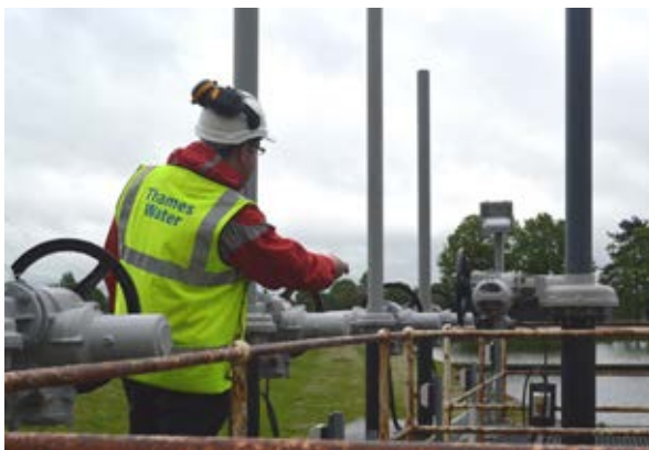
David West, Thames Water's West London Abstraction Engineer, uses the non-intrusive setting tool to operate an IQ3 actuator at the upgraded reservoir inlet site.
