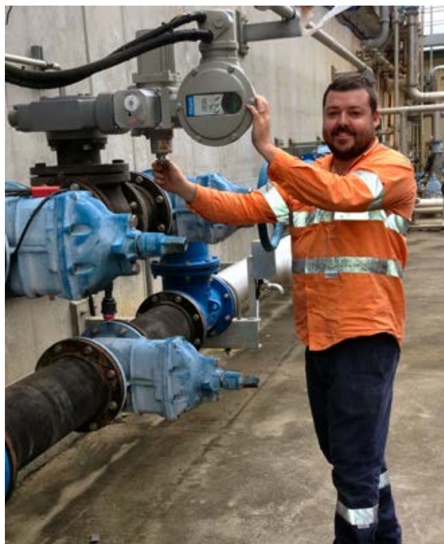
Photocaption: A SIPOS Aktorik actuator and gearbox combination supports essential sewage control processes at Brooklyn STP.
