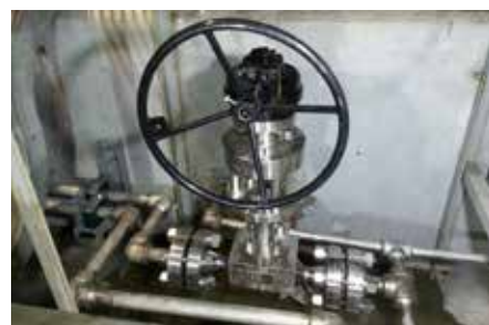
Bestobell Marine is currently the only manufacturer of high pressure cryogenic Globe valves for use in ships' gas fuelled engines
