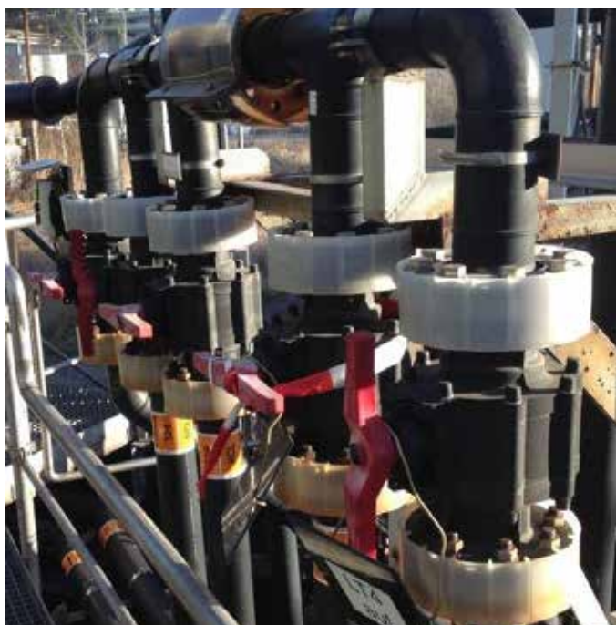
HCL PROCESS: Often lined valves are specified for use on high concentrated acids. GRPP valves offer an effective solution
