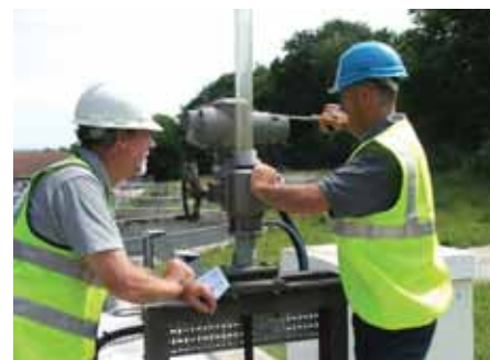
Figure 4: “Plug-and-play” components greatly reduce the amount of site work needed to install and commission motor operated valves.
