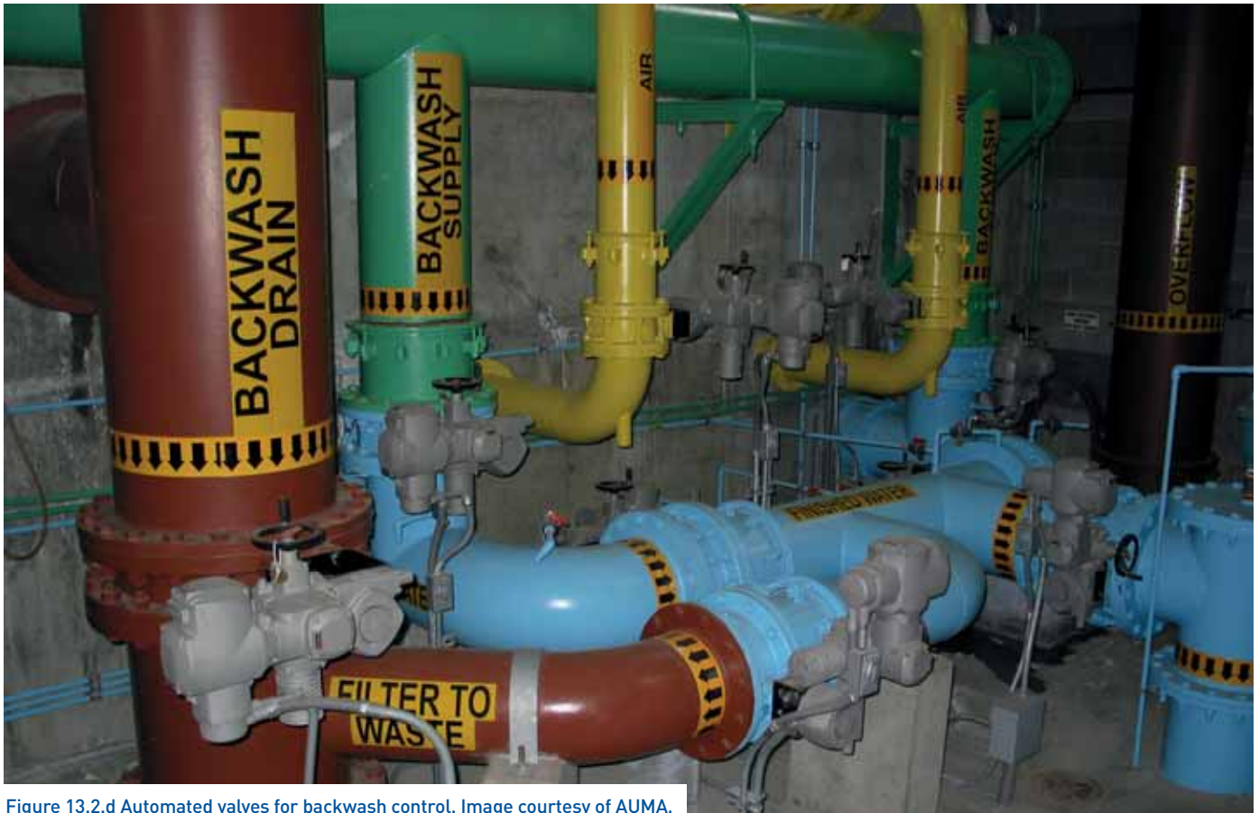
Figure 13.2.d Automated valves for backwash control. Image courtesy of AUMA.
