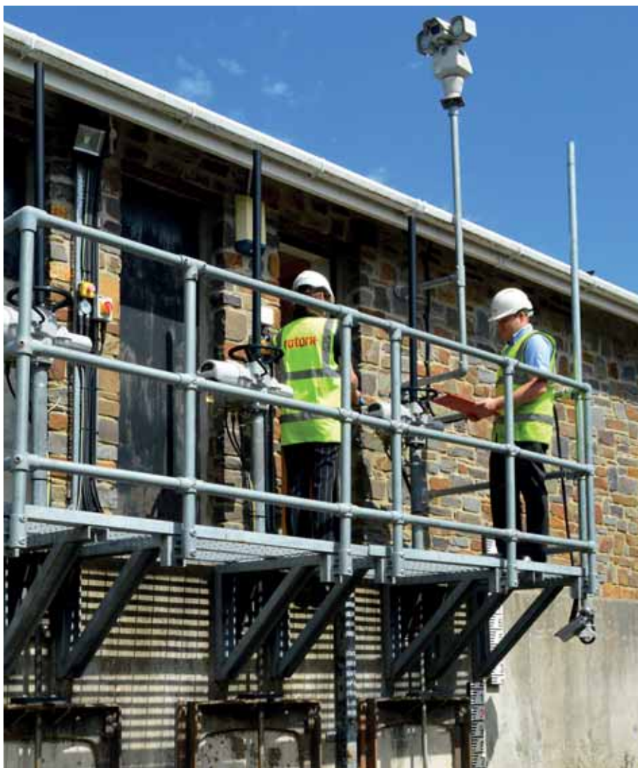
New Rotork IQ actuators installed on the flushing penstocks. The level sensor that controls the operation of the actuators via the PLC is situated in the downpipe installed between the back two penstocks. Two of the site's CCTV installations for remote visual monitoring of the river can also be seen.
